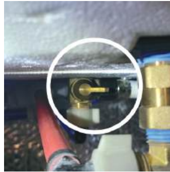
Water Heater Bypassed
