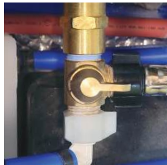
Water Heater Bypassed
