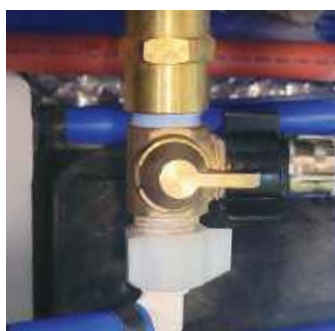
Water Heater Bypassed
