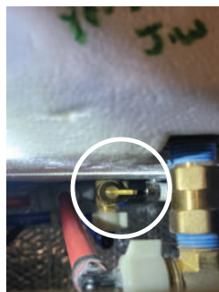
Water Heater Bypassed (does not allow water into water heater)
