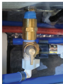
Valve Open (allows water into water heater)
