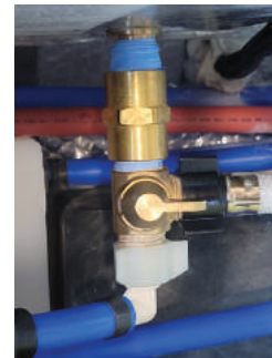
Water Heater Bypassed (does not allow water into water heater)
