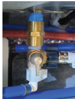
Valve Open (allows water into water heater)
